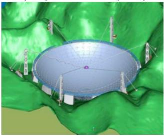
Composed of 4,600 panels, the spherical instrument's highly sensitive passive radar will also be of service in monitoring satellites and space debris, which will be a benefit to China's ambitious space program.
